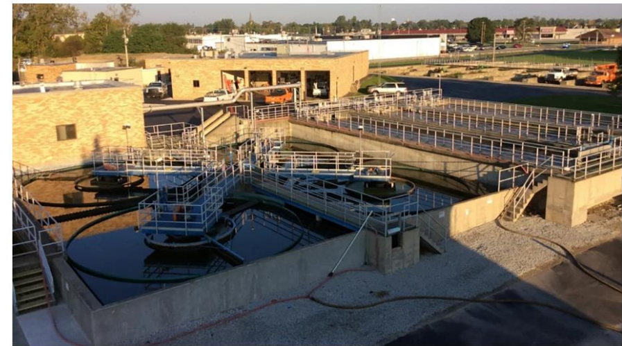
The Tipton, Indiana, wastewater treatment plant. From Tipton Municipal Utilities
